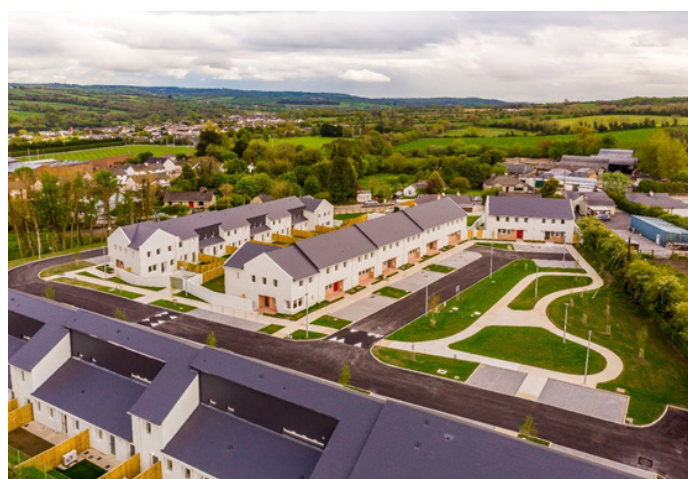
Aerial view of completed scheme at Glebeside, Castlecomer 33 units (KCC direct build)
