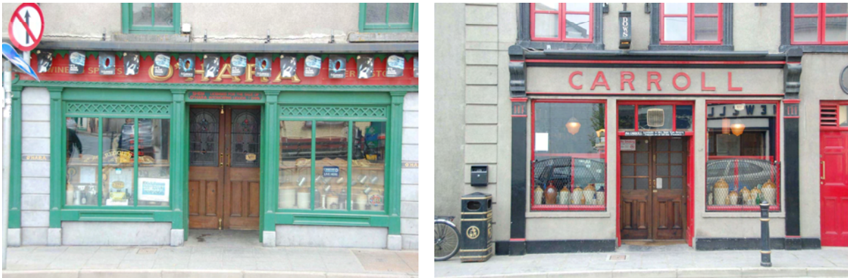
Examples of traditional shopfronts in Thomastown
