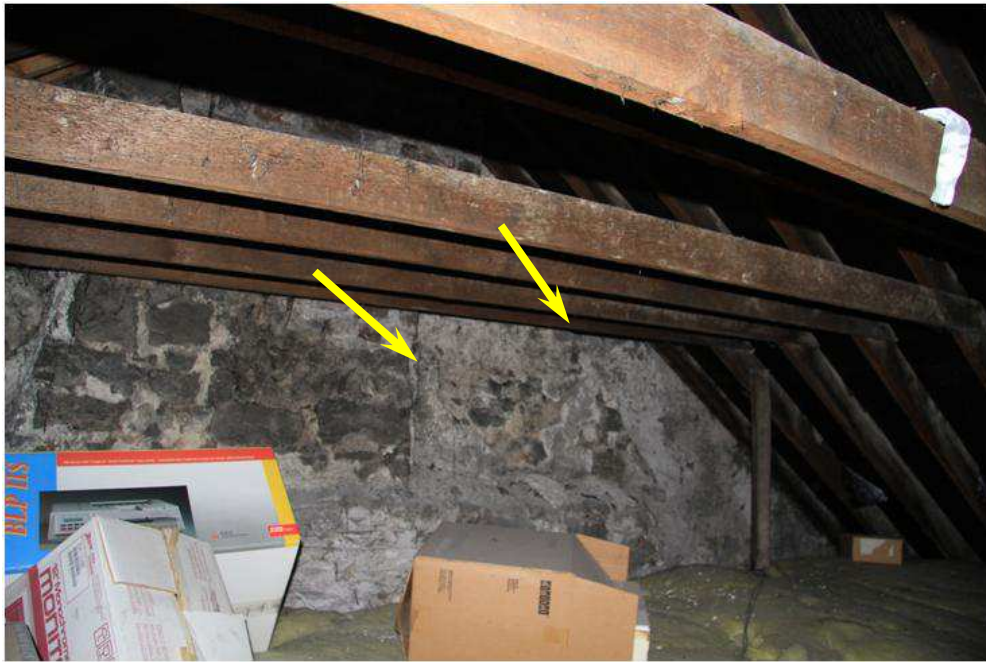
Plate 18: Party wall with number 76 at attic level - front
