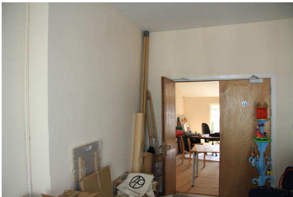
Plate 31: View to rear of room over passageway
