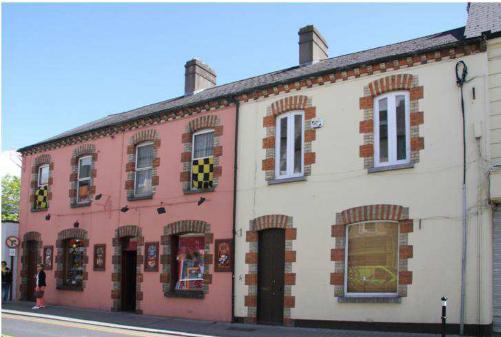
Figure 7: 73, 74 and 75 John Street Lower
