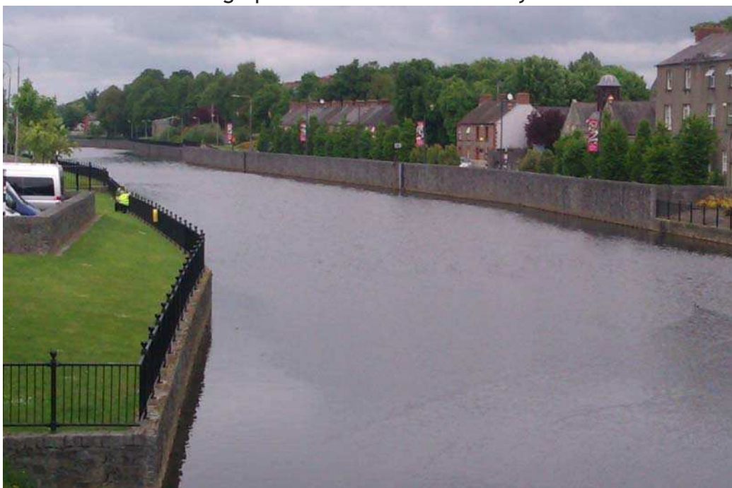
Photograph 6: Flood defences Upstream on the River Nore
