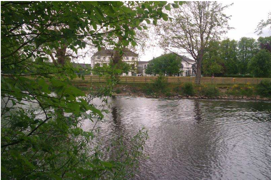
Photograph 1 & 2: Council Offices from River
