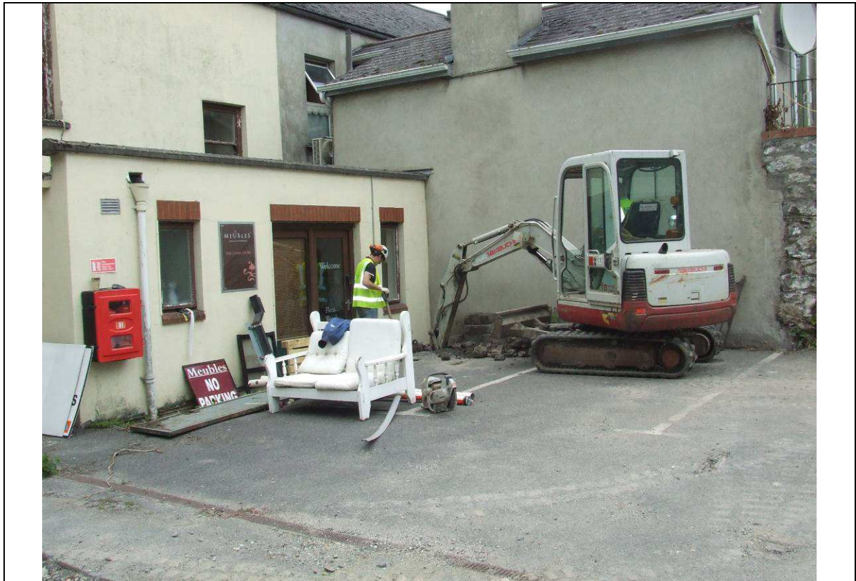
Plate 20: Trial Pit 1, under excavation, looking northwest.
