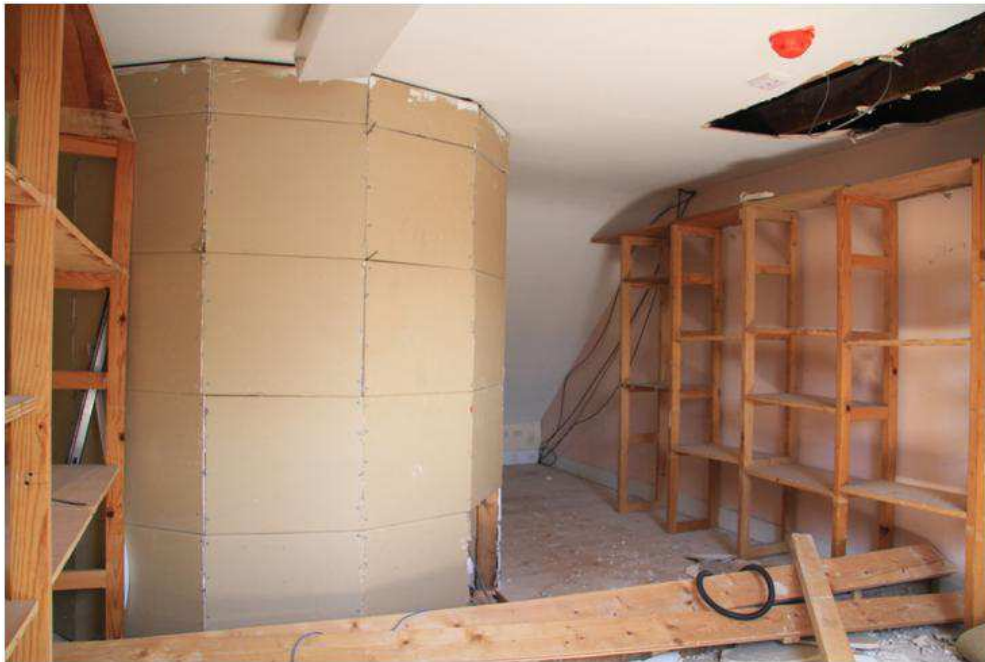
Plate 36: Space at attic level above passageway from street.
