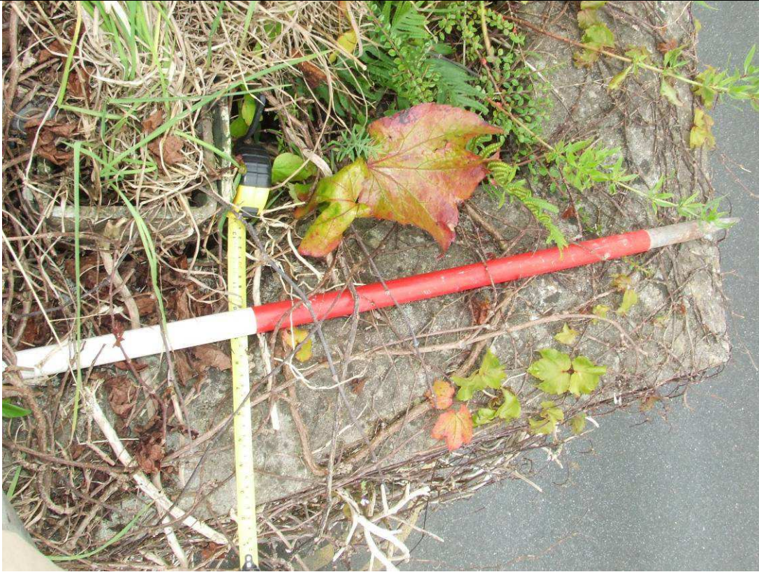
Plate 3: View of northeast corner of masonry wall from above. Note the corner of the Arts Building (top left).
