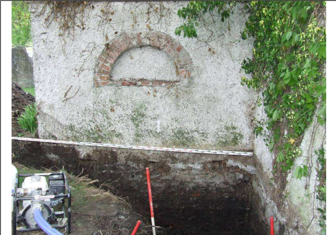
Plate 7: Upper mill wall C2, Trench II, Collegetownland (Phase 1A), looking south.
