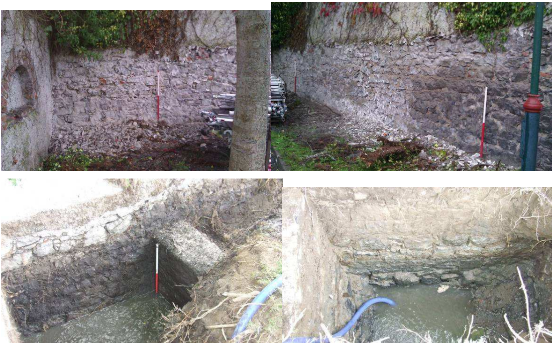
Plate 7: Composite views of masonry wall looking west, with plaster removed and under excavation.
