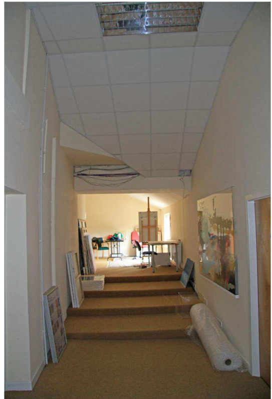
Plate 34: View along corridor with main building at left
