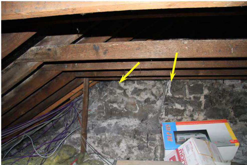
Plate 19: Party wall with number 76 at attic level – rear
