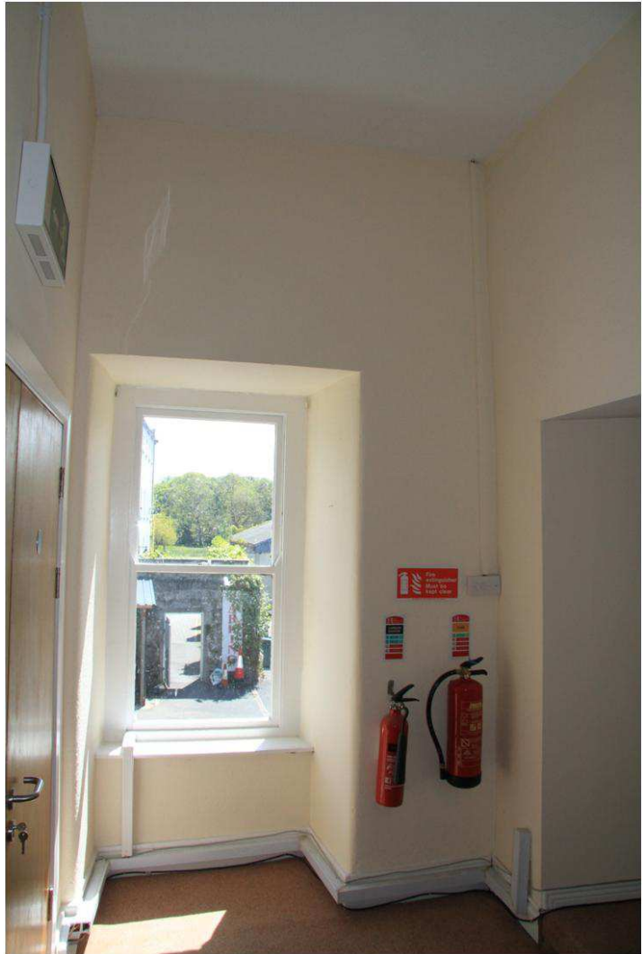
Plate 14: Window in corridor, with door to number 76 at right
