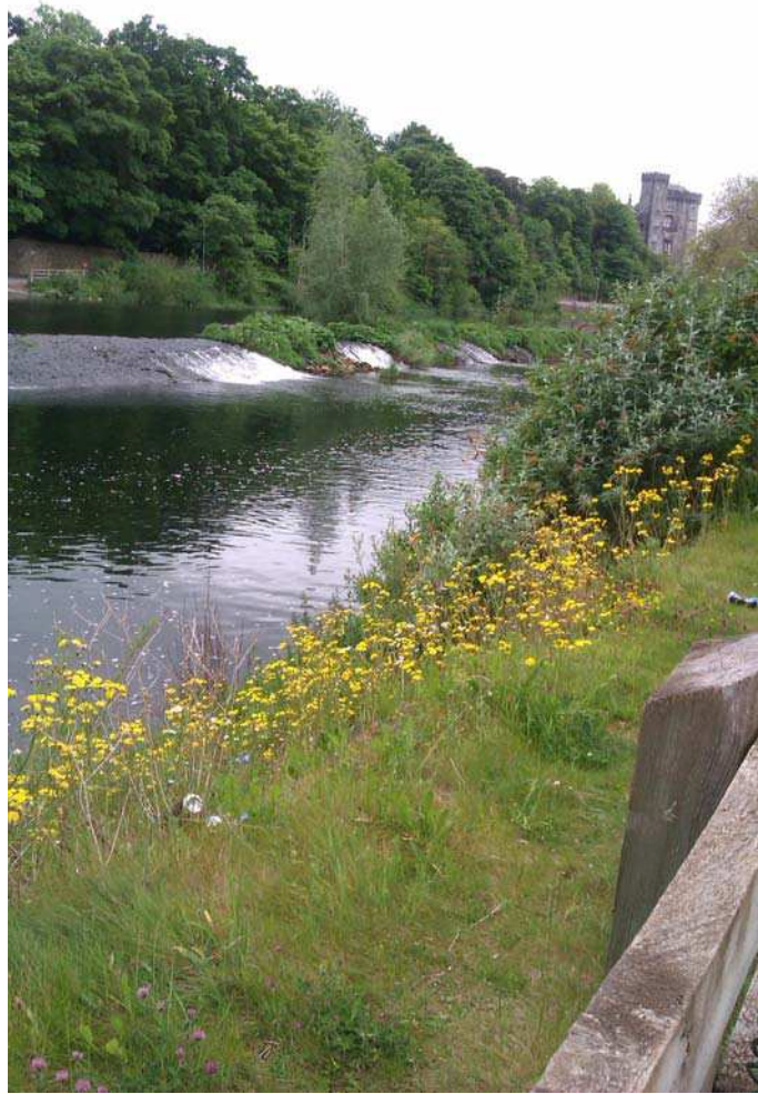
Photograph 5: Weir in River Nore by Site
