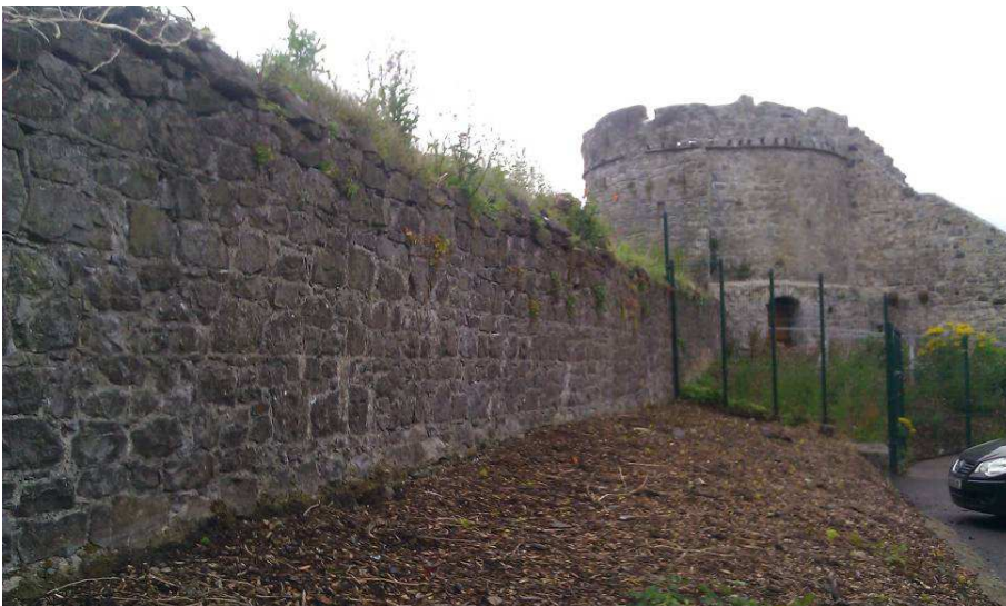
Plate 5: View south of Talbot's Tower and extant town defensive wall, on Ormonde road, Kilkenny.
