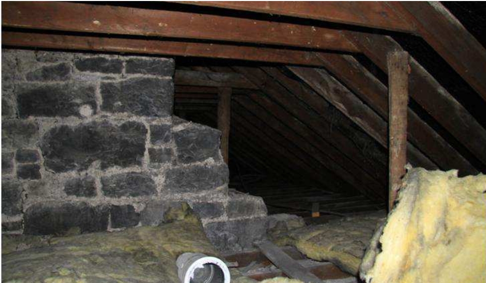
Plate 16: Party wall with number 74 at attic level – rear
