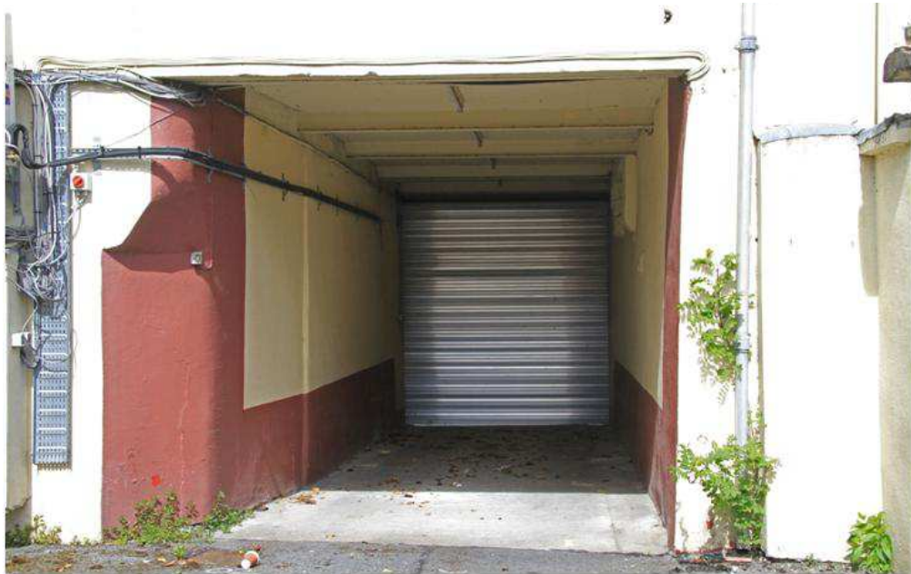
Plate 6: Access from street
