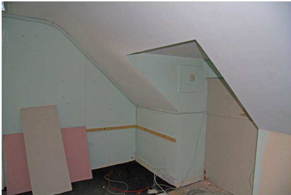
Plate 40: Rear office at south-western end of attic floor
