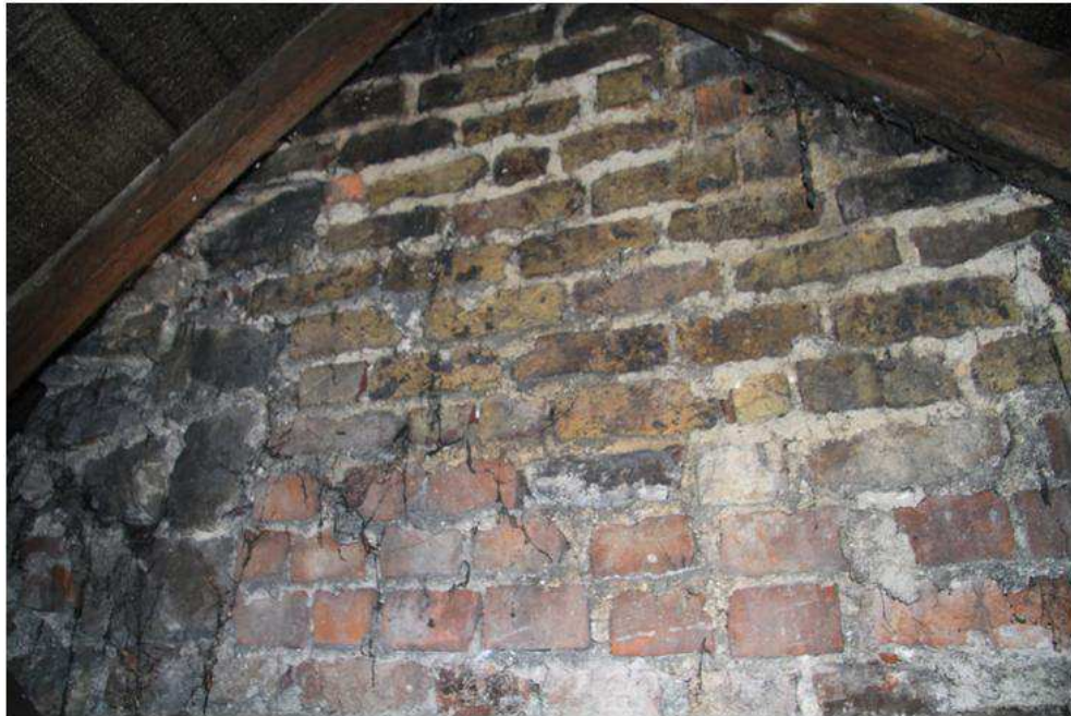
Plate 41: Central section at top of party wall between numbers 76 and 75
