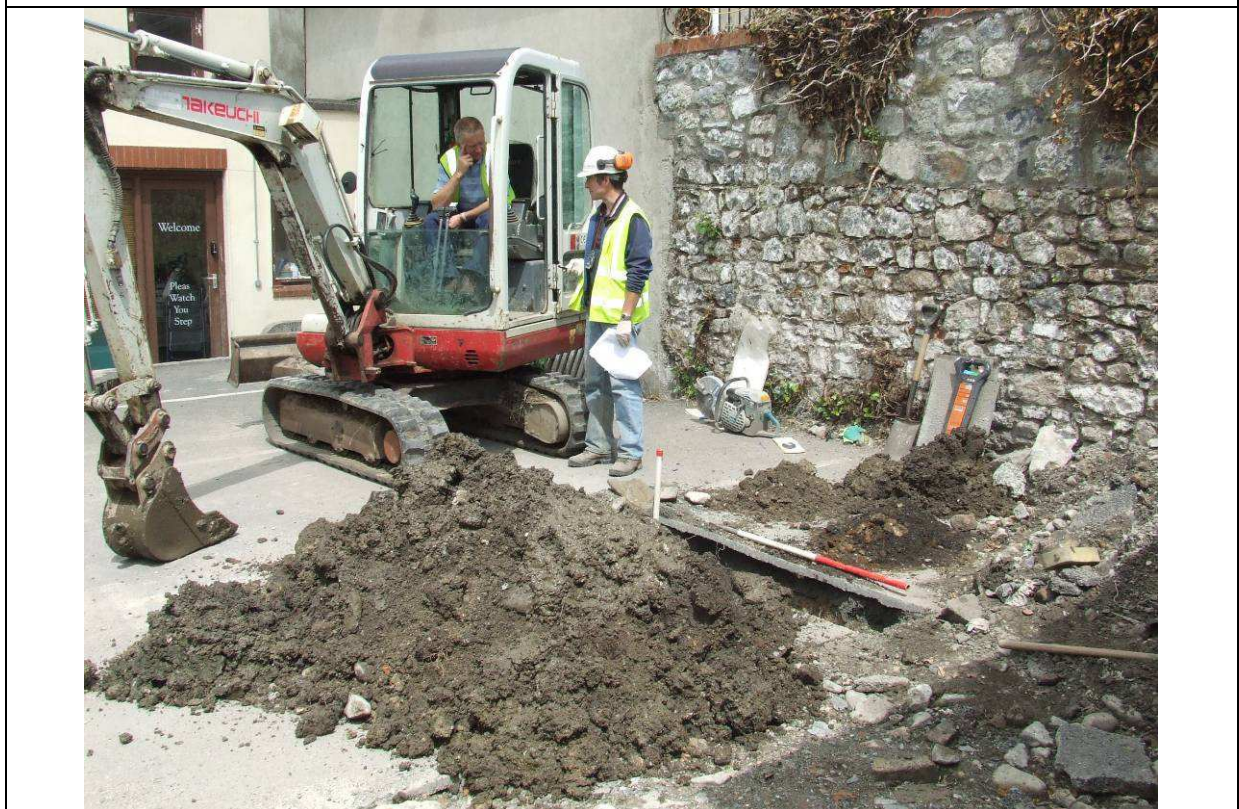
Plate 21: Trial Pit 2, under excavation, looking northwest.
