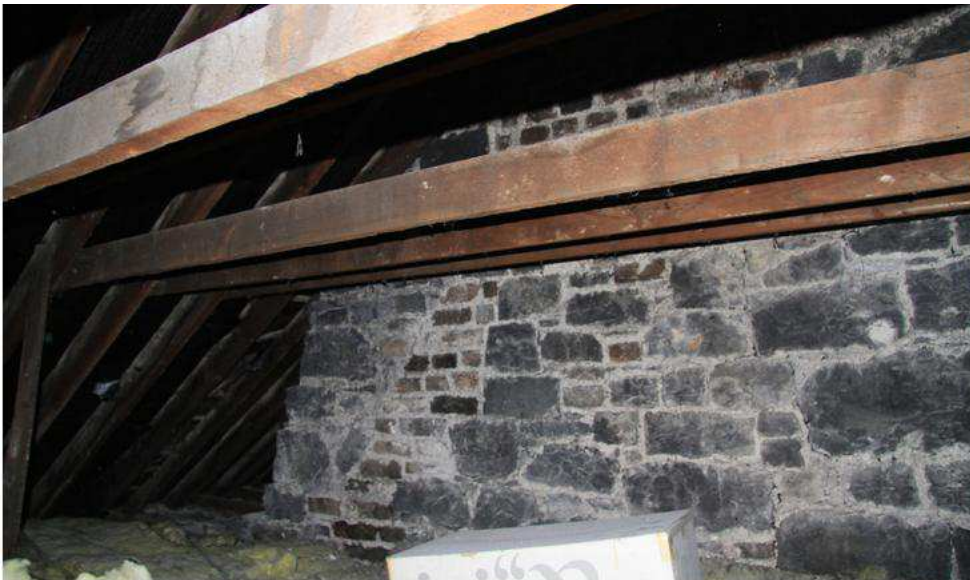
Plate 17: Party wall with number 74 at attic level – front
